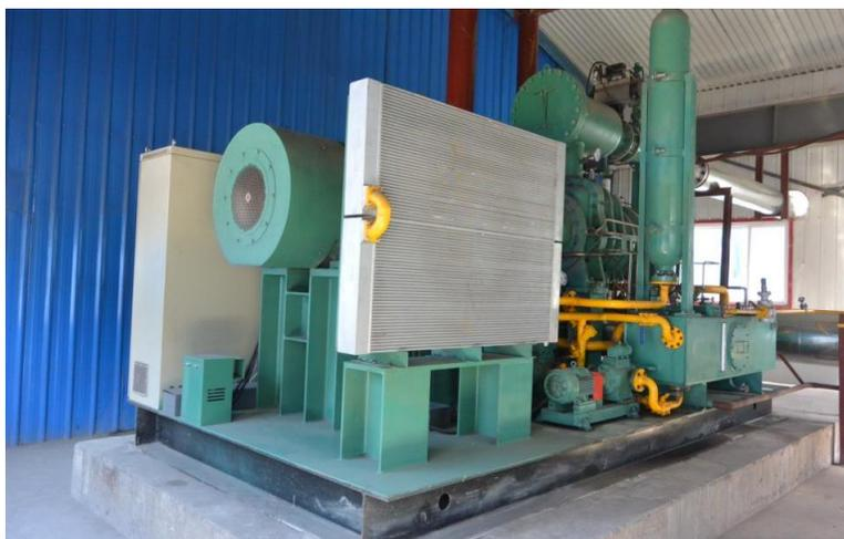
**Fig. 2:** steam expander KES600 installed at Tianfeng power plant No. 1
